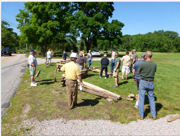
Split-rail fence construction at Homestead
